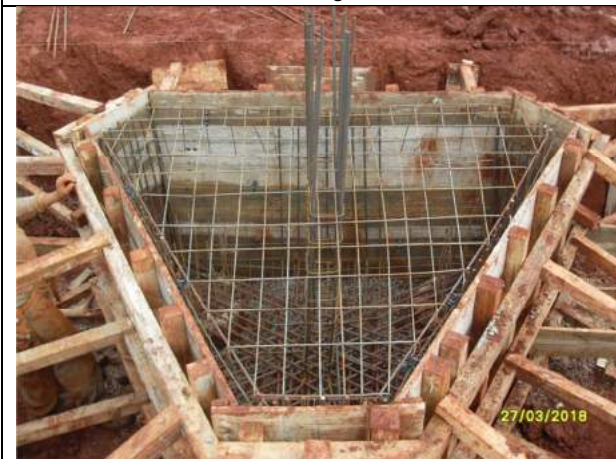
Foto 03 – Bloco triangular a concretar
